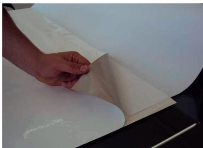
**Step 5:** Fold back the SAV to "encapsulate" the varitex between the SAV and the backing paper.
